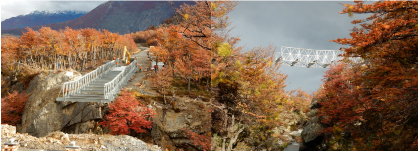
Launching of a panel bridge
