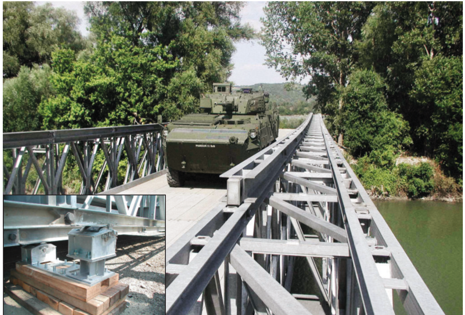
The panel bridge in Klosterneuburg near Vienna was built jointly with the Austrian Federal Armed Forces.
